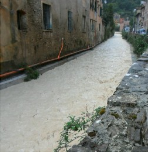
Above: the Carriona river after flooding.
